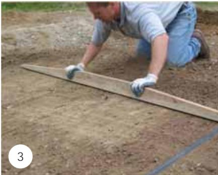
**Preparing your Base:** For patios and walkways minimum base thickness is 4". For driveways please consult your paver supplier for proper installation. Like compaction of your soil, subgrade compaction on your gravel base in 2" lifts.
