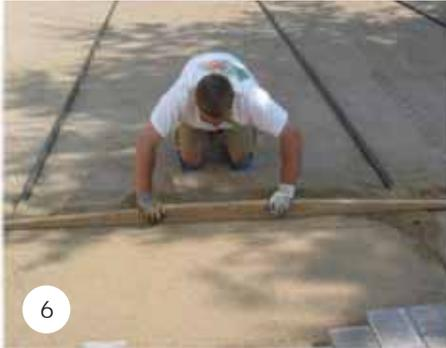
**Placing the Bedding Sand:** Concrete sand is recommended and should be spread and leveled to a consistent thickness of 1" and 1 1/2".
