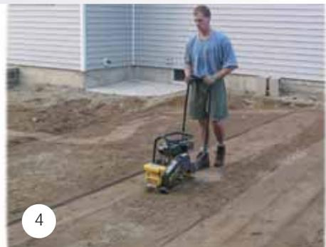
**Building your Edge Restraints:** Edge restraints are key to your installation. They provide lateral resistance which keeps your pavers from separating. Place your edge restraints on the compacted gravel base. Never place edging on the bedding sand. Secure the edging into the compacted gravel base using 10" spikes. Let the edging follow your patio or walkway perimeter design.
