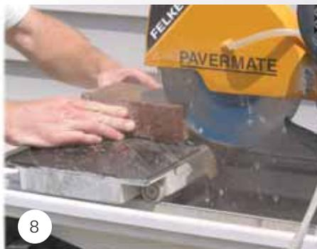
**Cutting the Pavers:** Cut pavers should be used to fill gaps along edge restraints.
